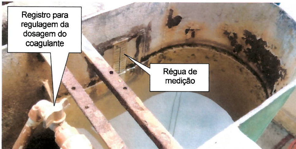
Vertedouro triangular
