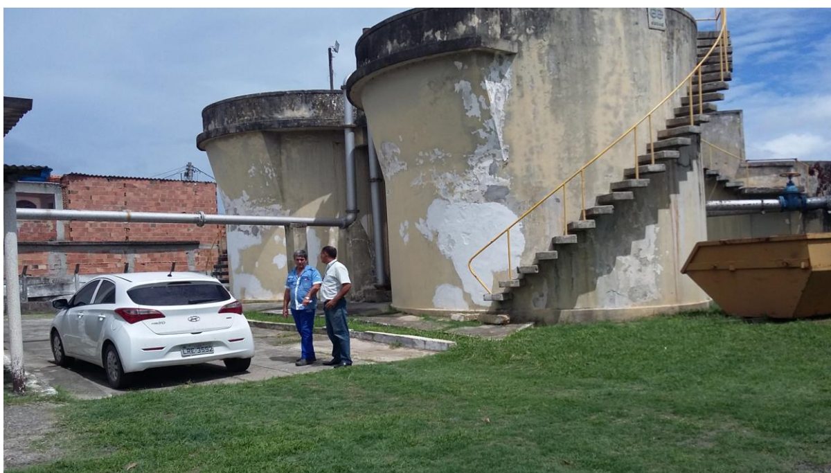
TANQUES IMHOOF - VISTA GERAL
