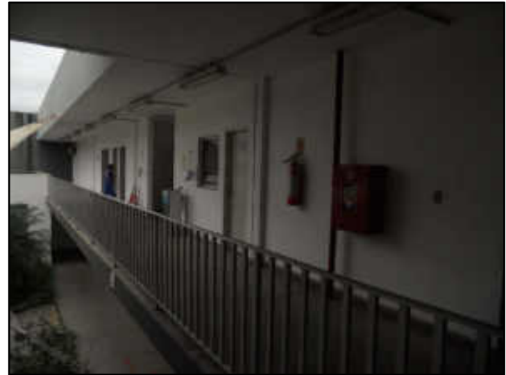
Corredor de acesso as salas
