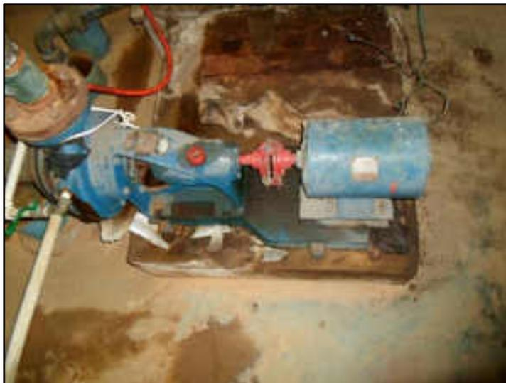
5.36.2. ETA VARRE-SAI - MOTOR ASSICRONICO TRIFASICO NA 5 CV 60 HZ 1700 RPM 220 380 440 V
